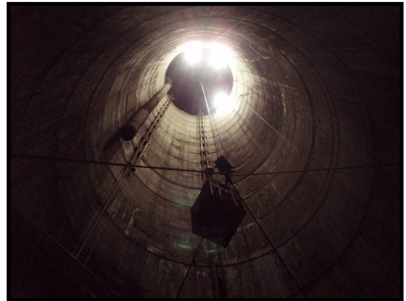
Access Shaft for Intake No. 3
